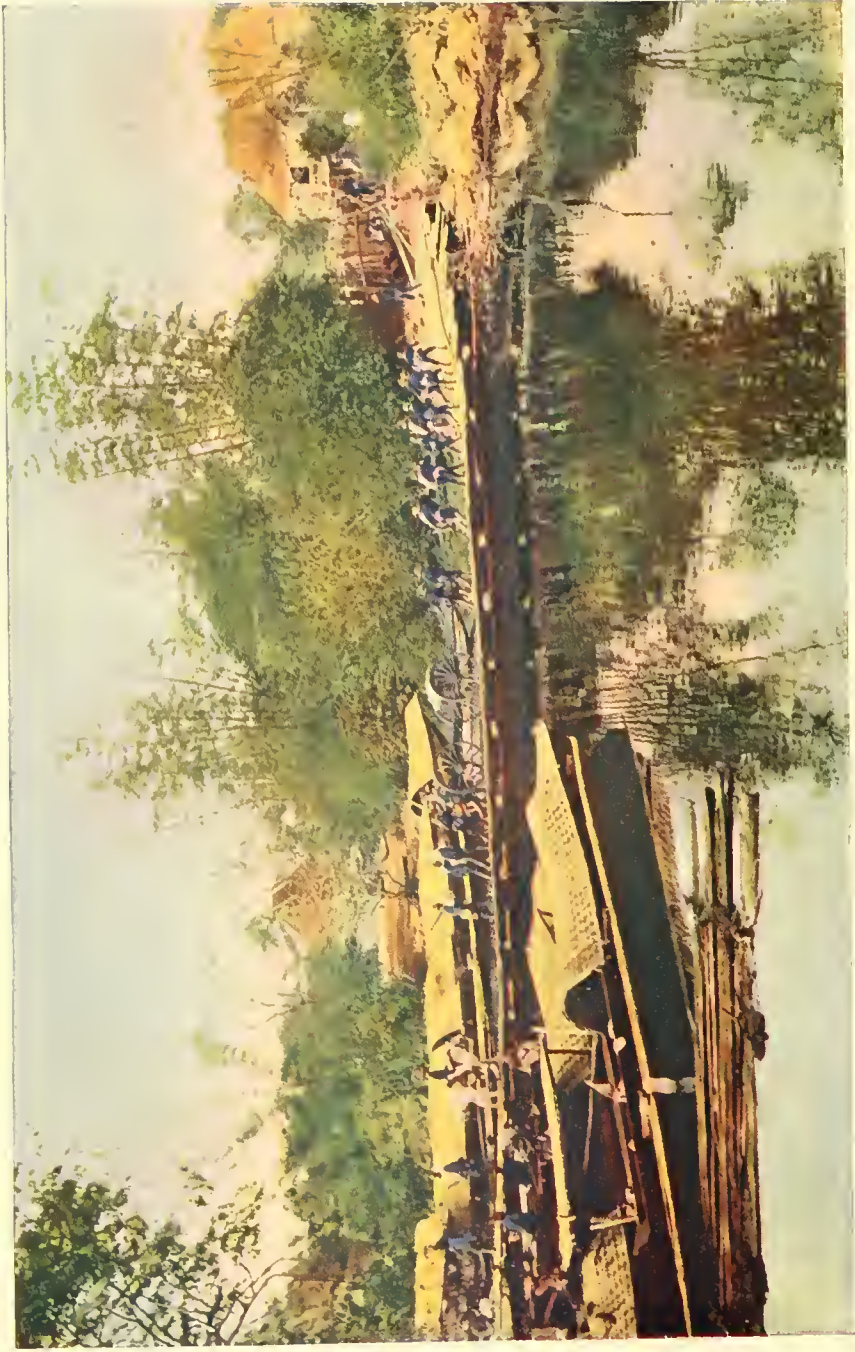
The American engineers usually had bridges ready as soon as they were needed. This was made in a few hours strong enough to allow the passage of artillery. The stream in this scene is known as the Bigan river.
